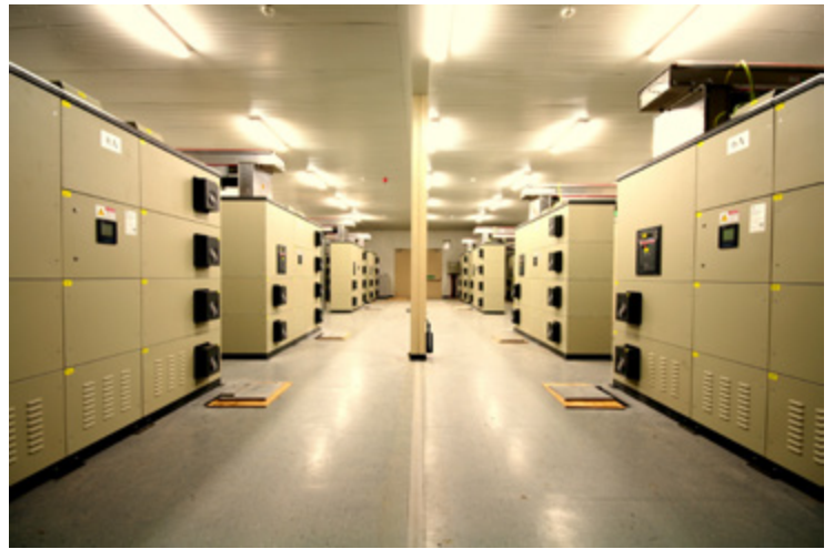
32MVAR Equalizer System installation at the substation
